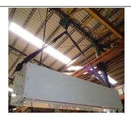
2. There are two round fitting-openings in the bottom, two sides of the curtain/motor box. Have the fixed bolt heads on the triangle plates fit the fitting openings, and then insert the bolts from the bottom.
