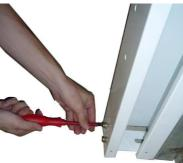
4. Install the infrared-sensor reflector on the lower left pillar. Insert the infrared sensor cord into the lower right pillar and, then, attach the infrared sensor. Place the cord in the cord-trough inside the right pillar.
