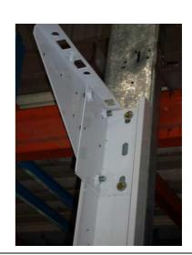
2. Attach the pillar-cover ground brackets with bolts or anchors.
