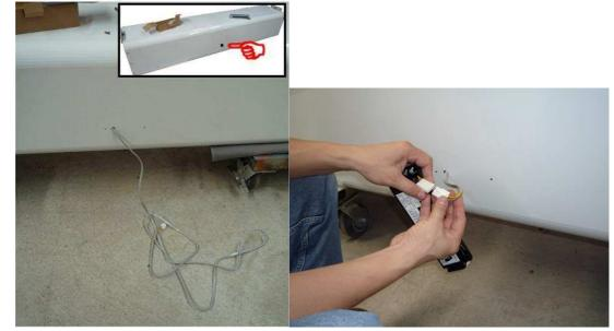
2. Attach the microwave sensor with screws on the front surface of the curtain/motor box, and then assemble the microwave sensor cover.
