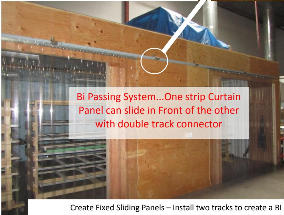
Bi Passing System...One strip Curtain Panel can slide in Front of the other with double track connector
